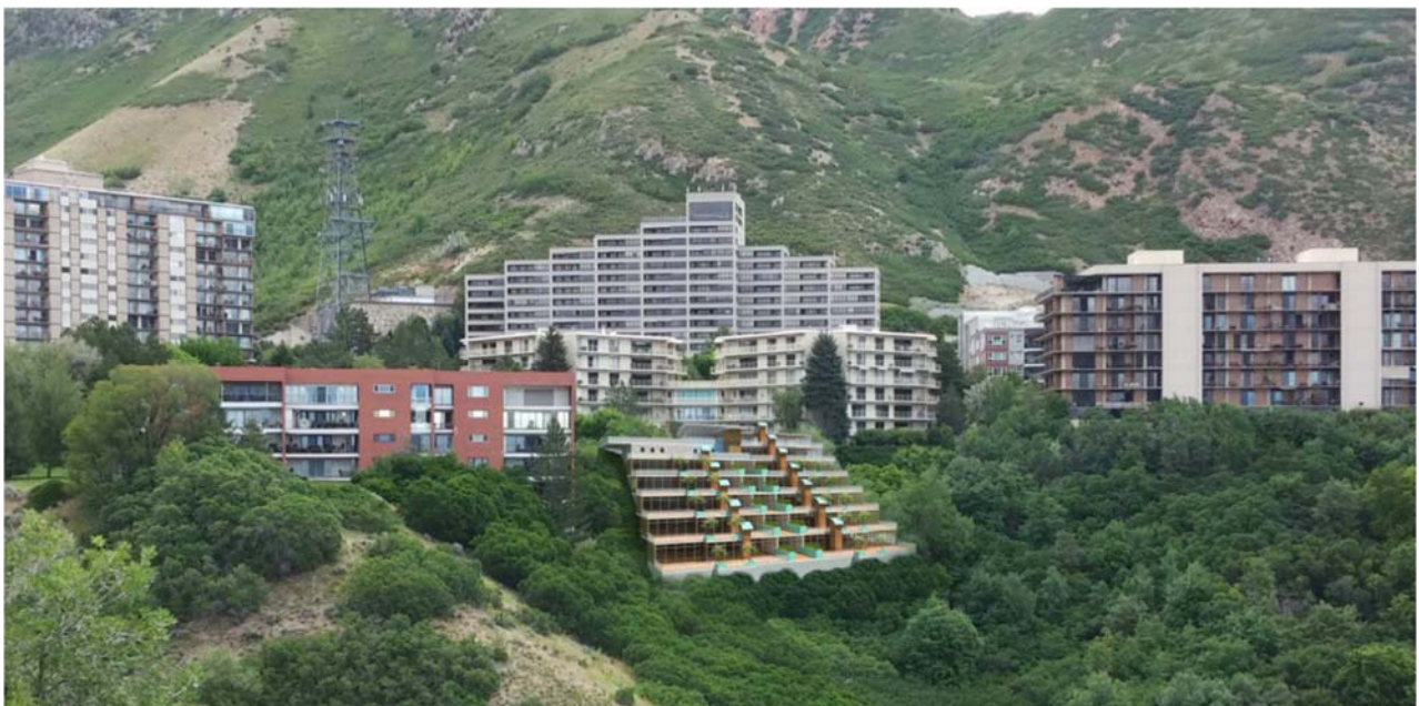
Rendering of the proposed structure (center of the image going down the slope)
